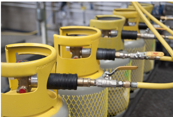
A-Gas Decant Facilities
